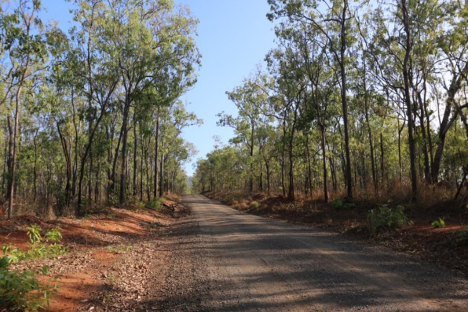
Davies Creek Road (Northern End), Davies Creek NP
